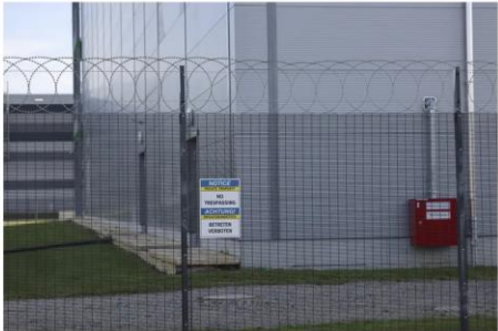
Security fencing around the Google Cloud data center ahead of its ceremonial opening in Hanau, Germany, on Friday, October 6th, 2023. Photo by Alex Kraus / Bloomberg via Getty Images
